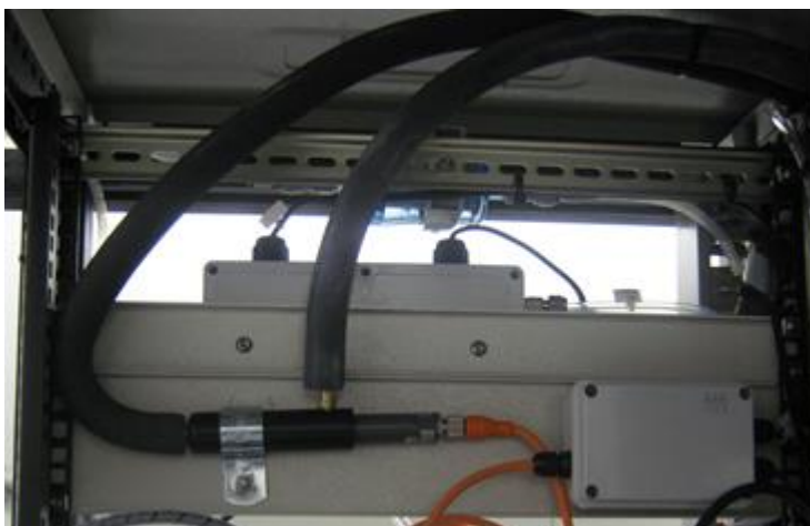
Figure 158 – Example of installed CO 2 Sensor
